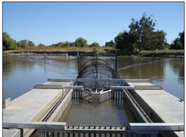
Fish will be collected using fyke nets installed upstream of the HFB. Fyke nets used in the mainstem river are constructed of two 150 ft long, 6-ft tall, 1.5 inch #15 treated nylon wingwalls funneled to a 6ft x 6ft collection
