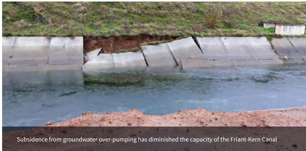
Subsidence from groundwater over-pumping has diminished the capacity of the Friant-Kern Canal
