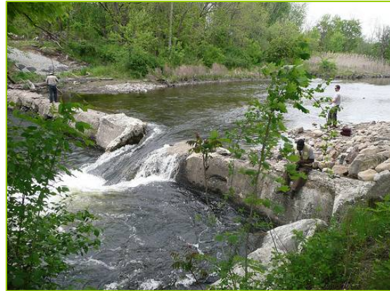
Figure 5-23. Spillway Notch
