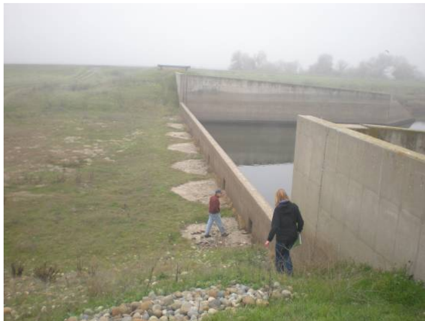
Figure 5-16. Mariposa Bypass Drop Structure
