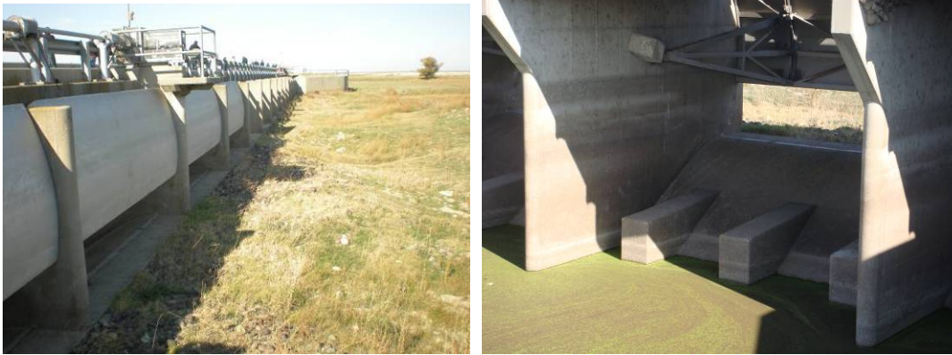
1 2 3 Figure 5-21. Mariposa Bypass Control Structure
