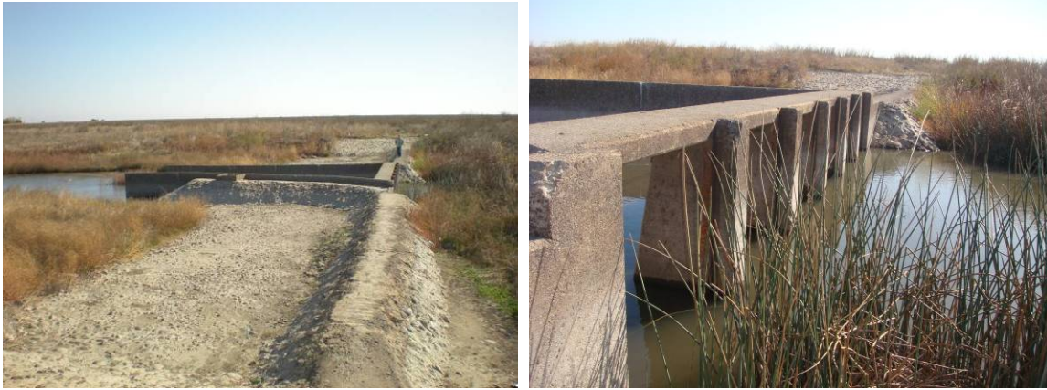
1 2 3 4 5 6 7 8 9 10 11 12 13 14 15 16 17 18 19 20 21 22 23 24 25 26 27 Figure 5-14. Sand Slough Control Structure
