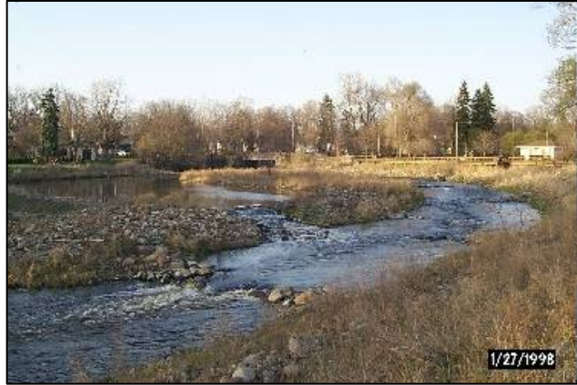
20 Figure 5-19. 21 Roughened Channel for Fish Passage
