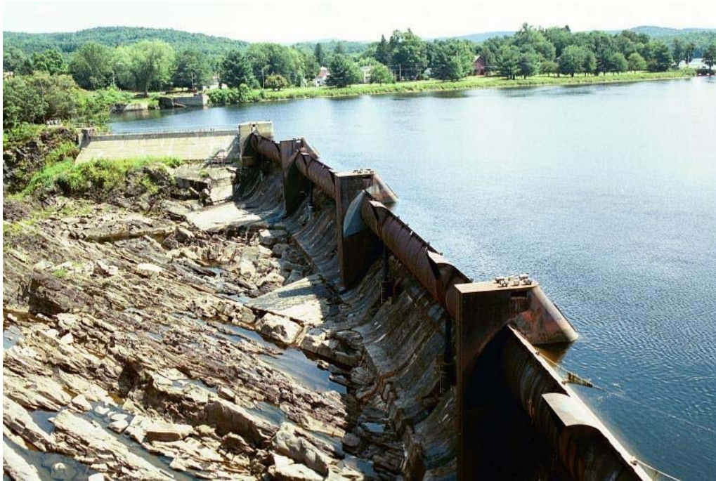
12 13 14 15 16 17 18 19 20 21 22 Figure 5-13. Hinged Crest Gate
