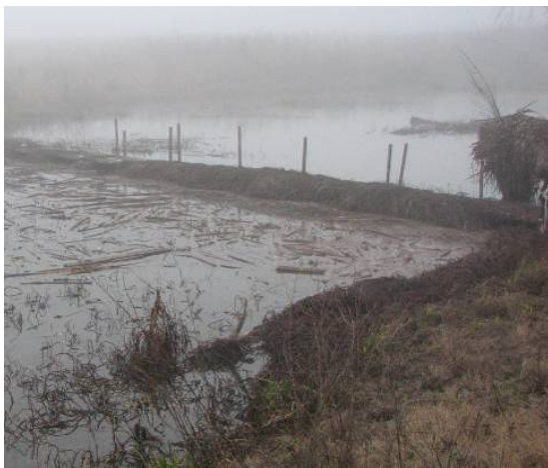
20 Figure 5-28. 21 Upper Weir
