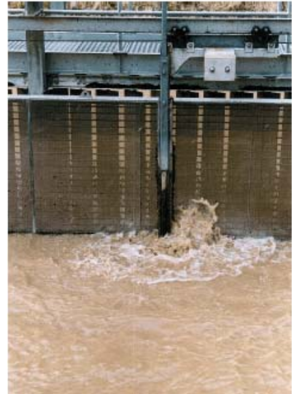
Figure 5-15. Vertical Fixed Flat Plate Screen
