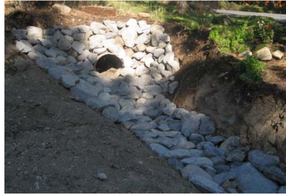
11 Figure 5-25. 12 Corrugated Steel Partially Buried Pipe 13 Arch Culvert
