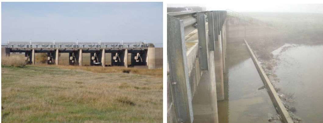
4 5 6 Figure 5-22. Eastside Bypass Control Structure
