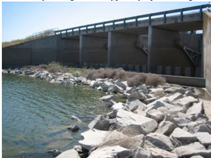
Chowchilla Bypass Control Structure outlet looking upstream
