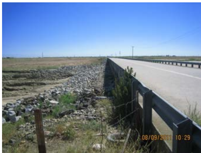
Avenue 21 Eastside Bypass downstream bridge crossing
