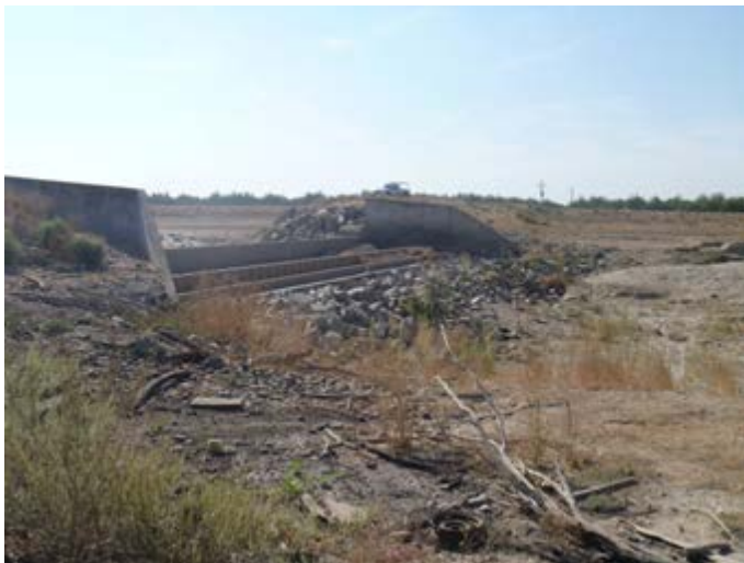
Drop 2 looking upstream within the Eastside Bypass
