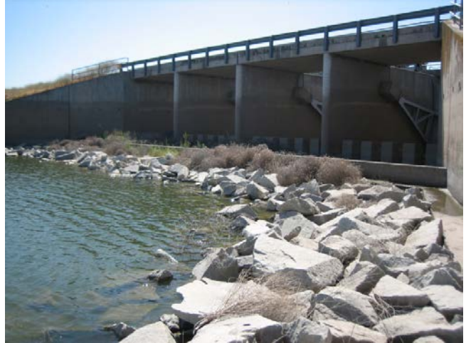
Photo 21_B. Downstream looking upstream from end of bay
