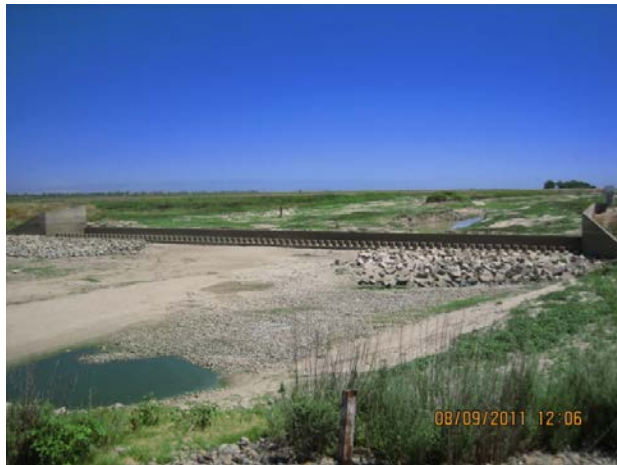
Photo 64_A. Drop 1 looking upstream
