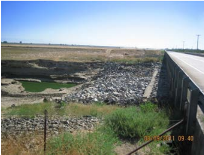
Avenue 18-1/2 Eastside Bypass downstream bridge crossing
