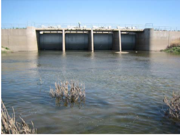
Photo 21_A. Structure, upstream looking downstream
