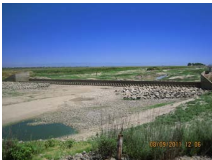
Drop 1 looking upstream within the Eastside Bypass
