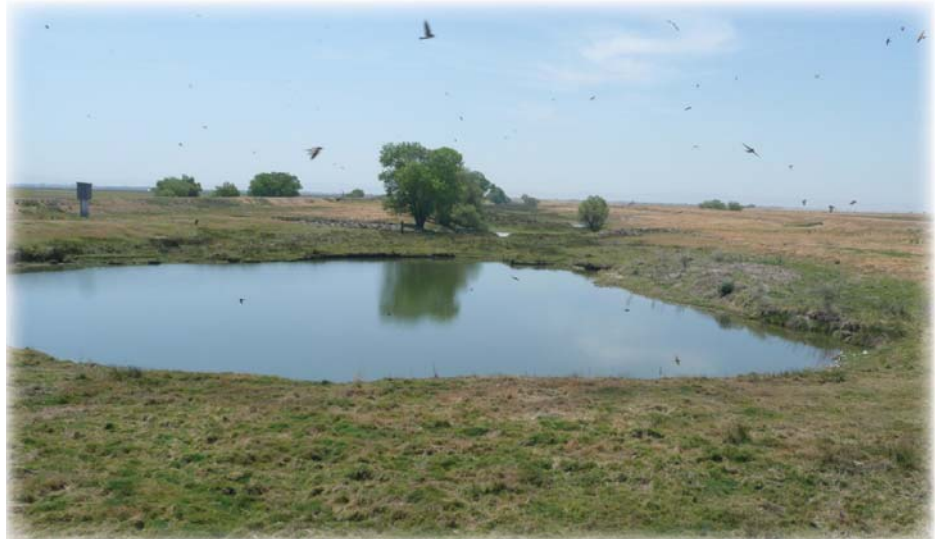
Viewed from the Mariposa Bypass Control Structure, the 3.3-mile-long Mariposa Bypass routes flood flows around Reach 4B1 of the San Joaquin River. The Mariposa Bypass typically receives the majority of Eastside Bypass flows when high flows are present in the Merced Streams Group.
