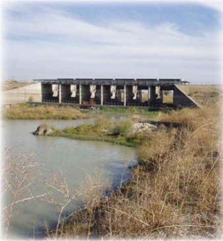
The Eastside Bypass Control Structure is one of two flood flow management structures that route San Joaquin River flows around all or a portion of Reach 4B. The Eastside Bypass is being considered as an option for routing of future Restoration Flows
