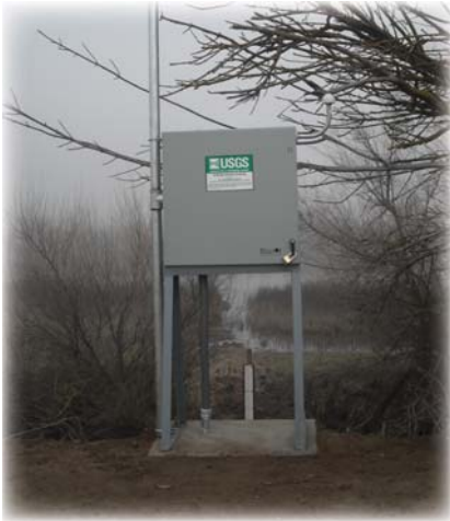
The newly installed San Mateo Gage
