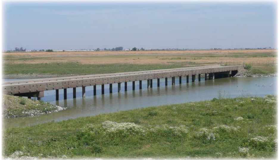
Private bridges in the Eastside Bypass are used by area landowners to transport farm machinery and equipment. Many of these bridges are inundated during flood operations.
