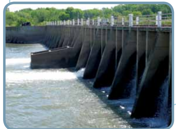
Mendota Dam at the Mendota Pool
