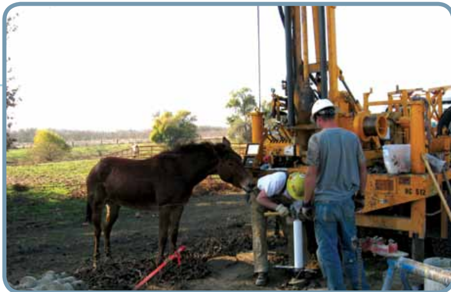
Reclamation's drill crew drilling one of the 34 monitoring wells installed in 2011, with a friendly mule taking a nibble. Reach 2A of the SJR. (12/7/2011)
