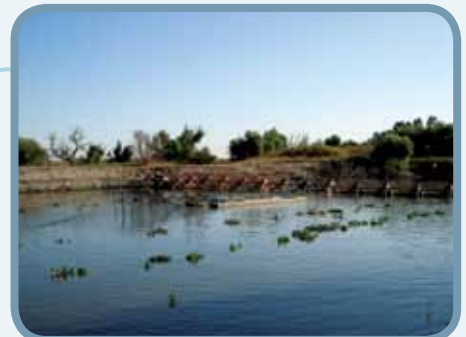
Hills Ferry Barrier
