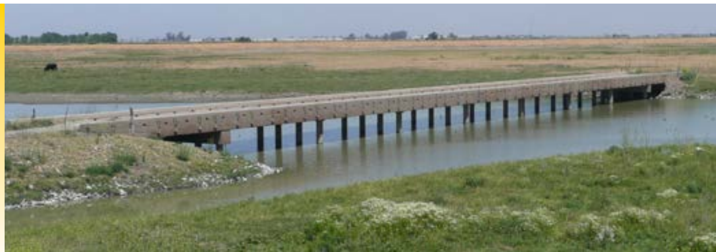
Eastside Bypass Bridge
