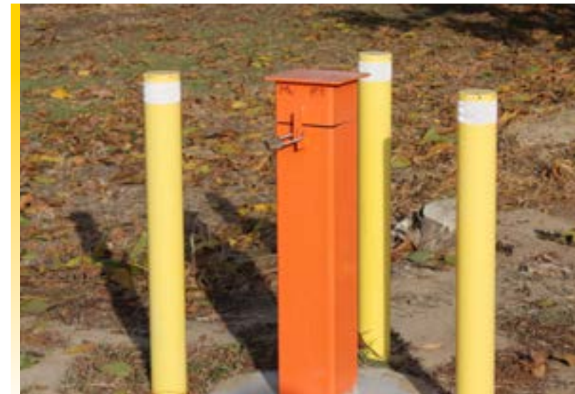
A newly installed monitoring well
