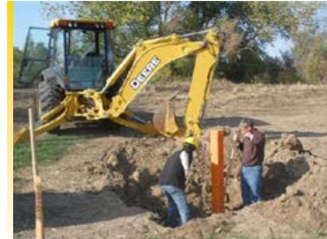
Installation of a monitoring well
