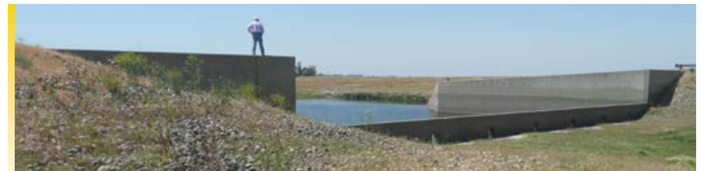
Mariposa Bypass Drop Structure
