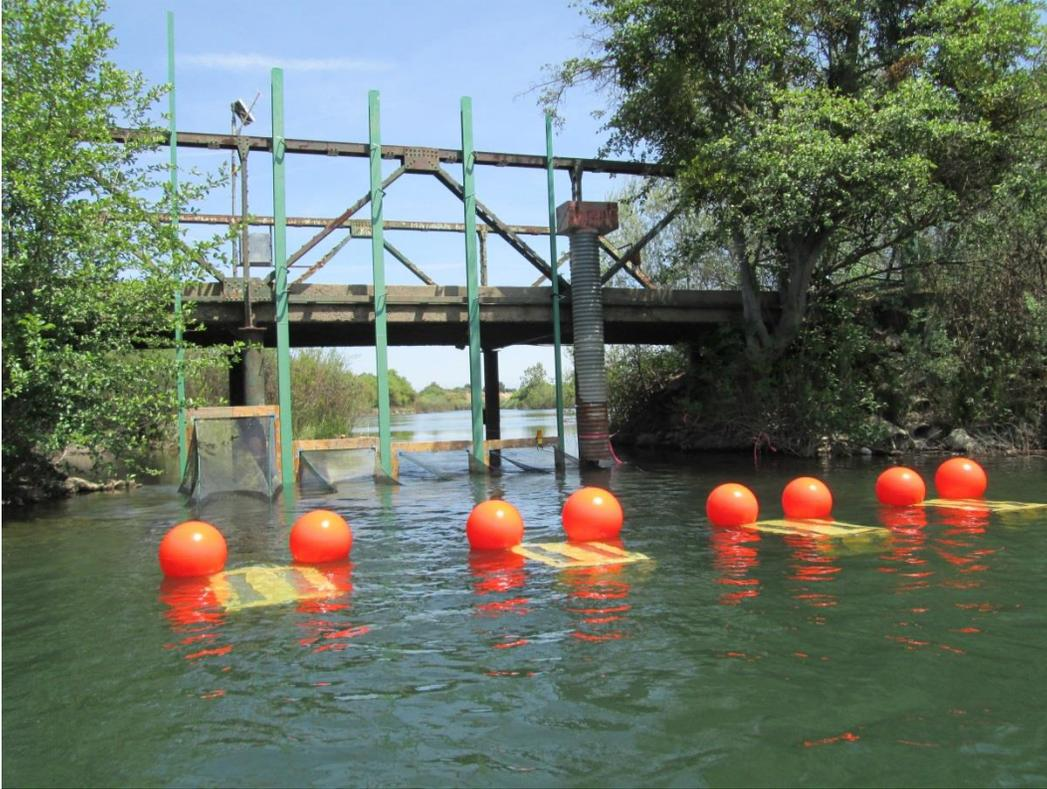
**Figure 3.–Entrainment-type nets temporarily installed on Donnie Bridge (River Mile 240.7) using aluminum channel clamped to existing structure. Collection boxes are attached to the terminal ends of the nets and free-floating using net buoys.**
