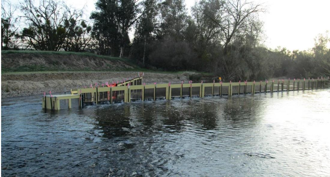
**Figure 1.–Temporary weir constructed at Scout Island (River Mile 250.1). Note the V-shaped opening facing upstream, designed to guide fish to the central collection box.**
