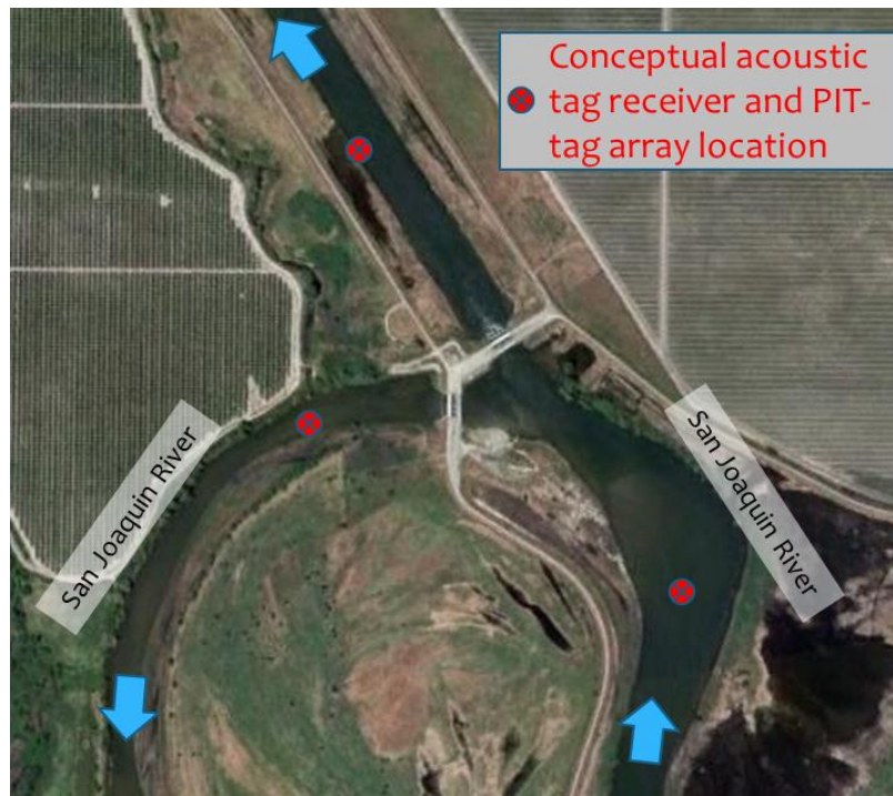
FIGURE 4: Conceptual placement of acoustic tag receivers to detect fish passage through the Chowchilla Bifurcation Structure.
