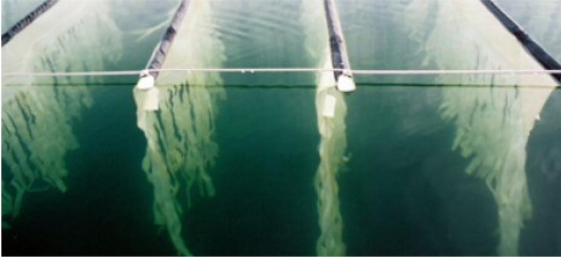
**Figure 6. Image of Aquamats suspended in pond.**
