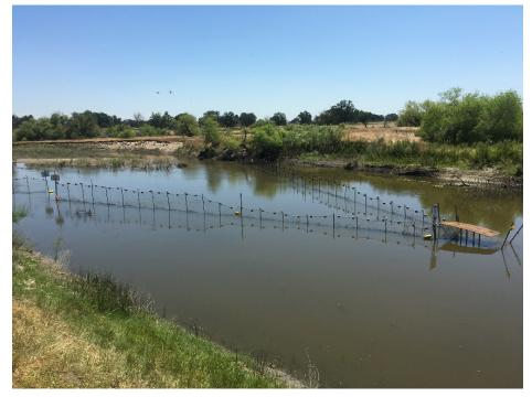
Figure 1: Net weir and fish monitoring facility at Hills Ferry in 2016.
