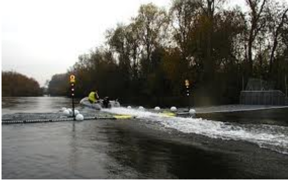
Figure 1. A motorized boat passing over a floating resistance weir.
