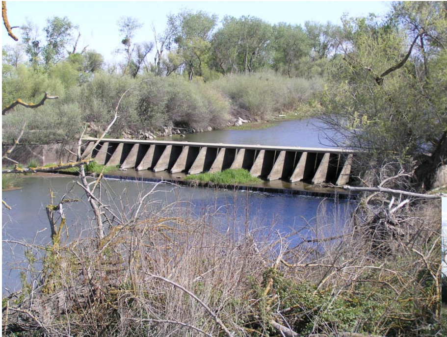
Sack Dam – Modify for fish passage
