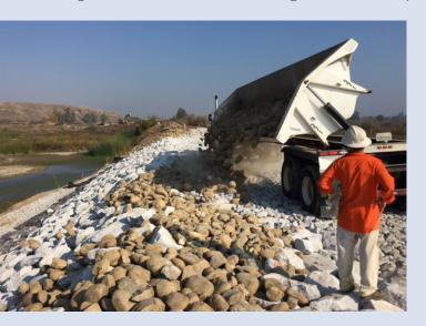
to isolate two gravel pit ponds from the river, and build a 250-foot rock structure for flood protection. Isolating the ponds will help salmon by keeping them in the river channel and away from predatory fish habitat in the ponds. The project also meets Program goals by improving access and allowing the Conservancy to more effectively manage their adjacent lands.
