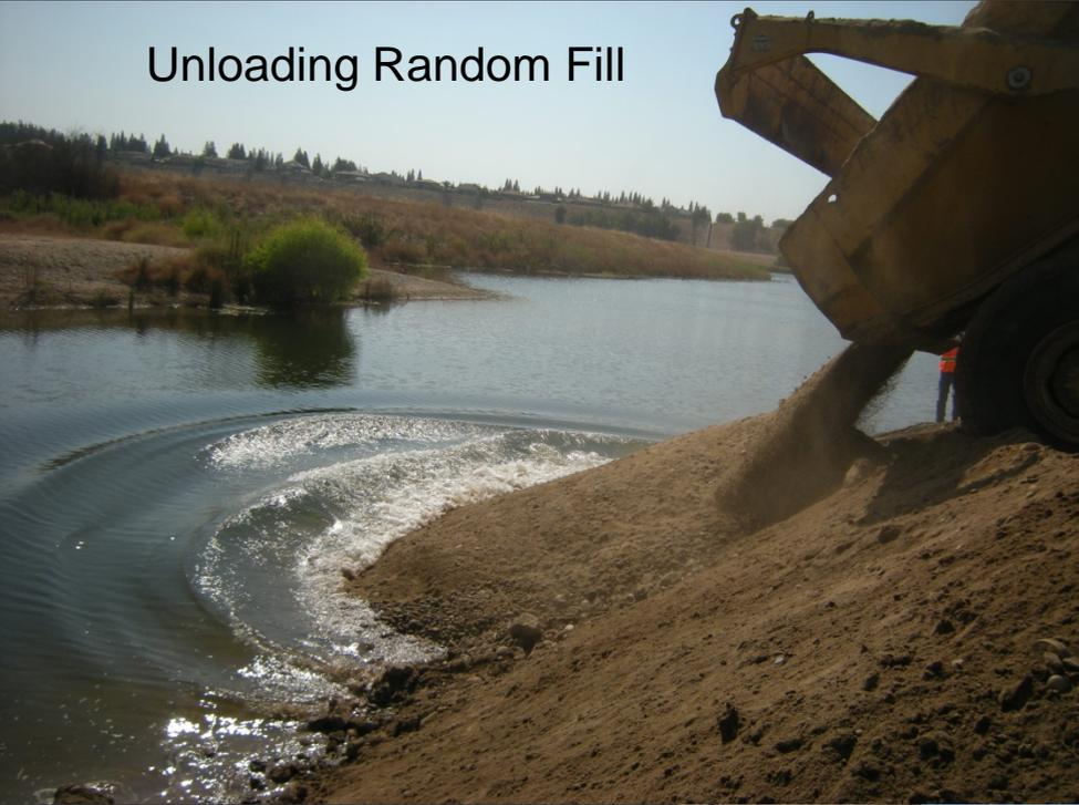
Filling Breach With Random Fill Below Water Surface
