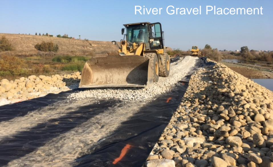
Geotextile Fabric Placement
