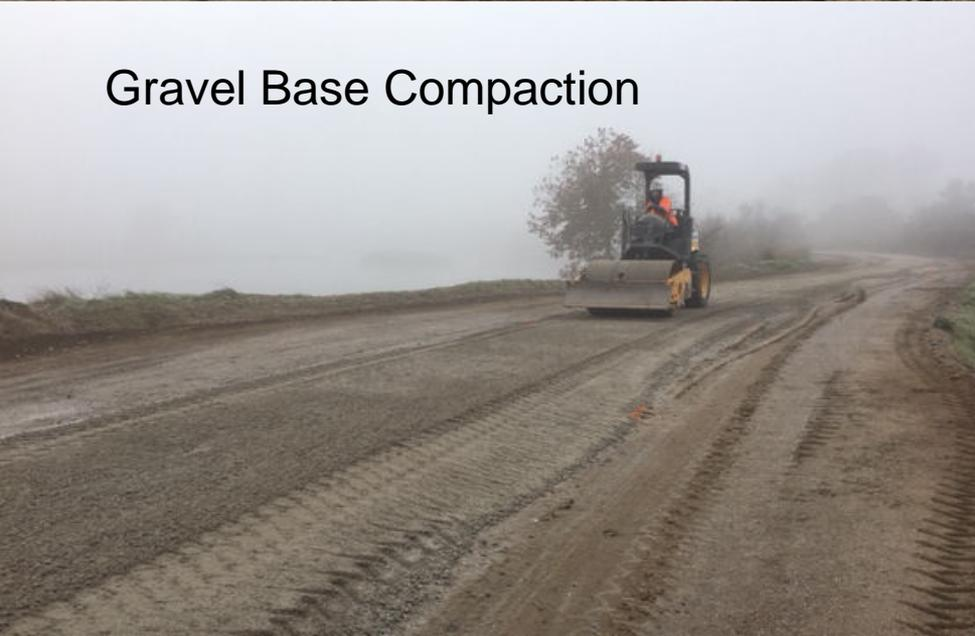
Gravel Base Placement on Top of Concrete Mat
