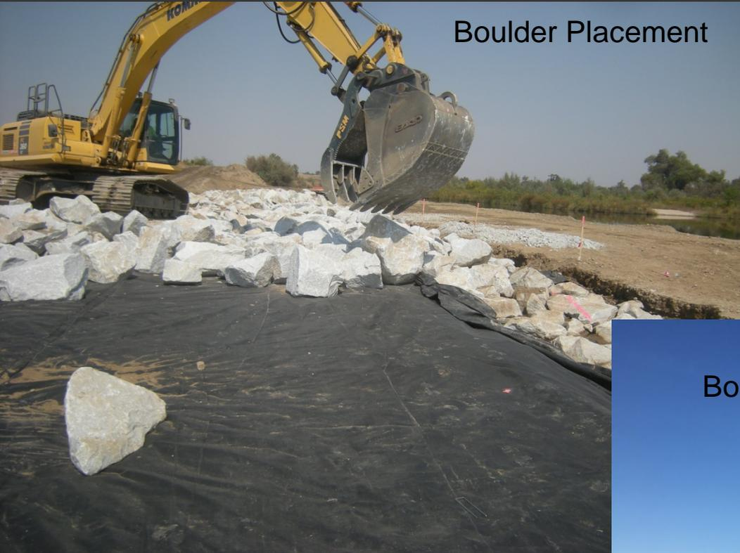
Boulder Placement and Compaction
