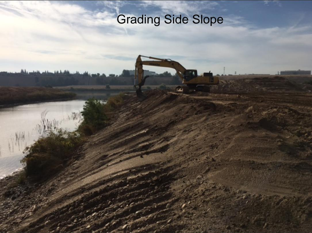
Re-Grading Side Slope to Generate More Material
