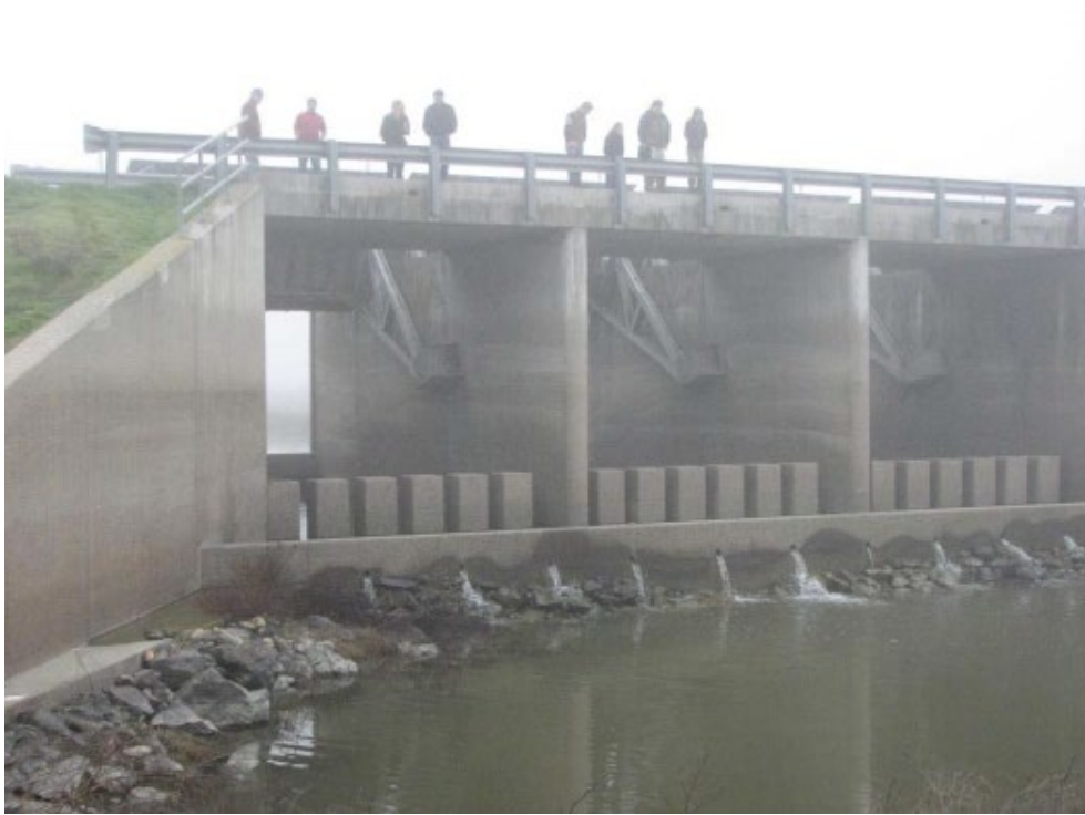
Figure G-6. Energy Dissipation Sills, Radial Arms, and Weep Holes within the Eastside Bypass Control Structure
