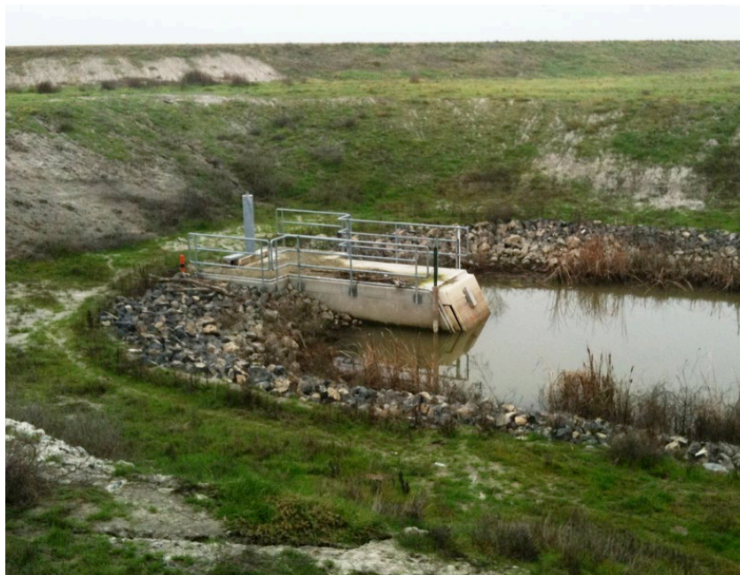
Figure G-1. Example of Pump Diversion within Reach 4B
