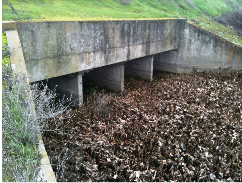
Figure G-2. Four Culverts Associated with the Reach 4B Headgates
