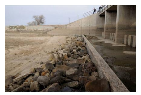
Figure 1-6 Concrete sill and bordering riprap along the downstream edge of the Chowchilla Bifurcation Structure in Reach 2B<sup>2</sup> (12/15/09)
