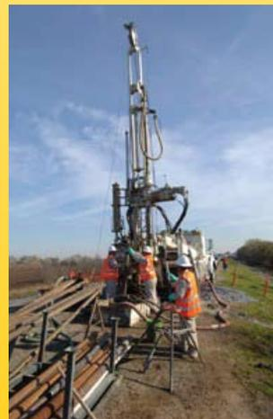
Geotechnical field crews drill borings to collect soil samples from a flood control levee.
