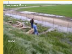
Levees are constructed on unstable foundations consisting of river sediment, mostly sand bars and sand strata. Even low flows can result in numerous sand boils and often levee failure in some reaches.
