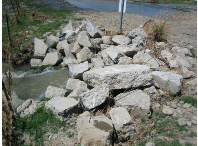
Photo 51\_E. Culvert inlet at flows less than 25 cfs
