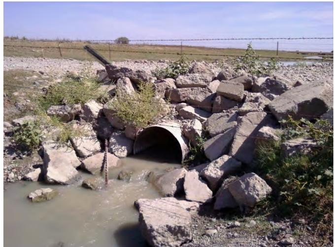
Photo 51\_G. Culvert for overflow channel
