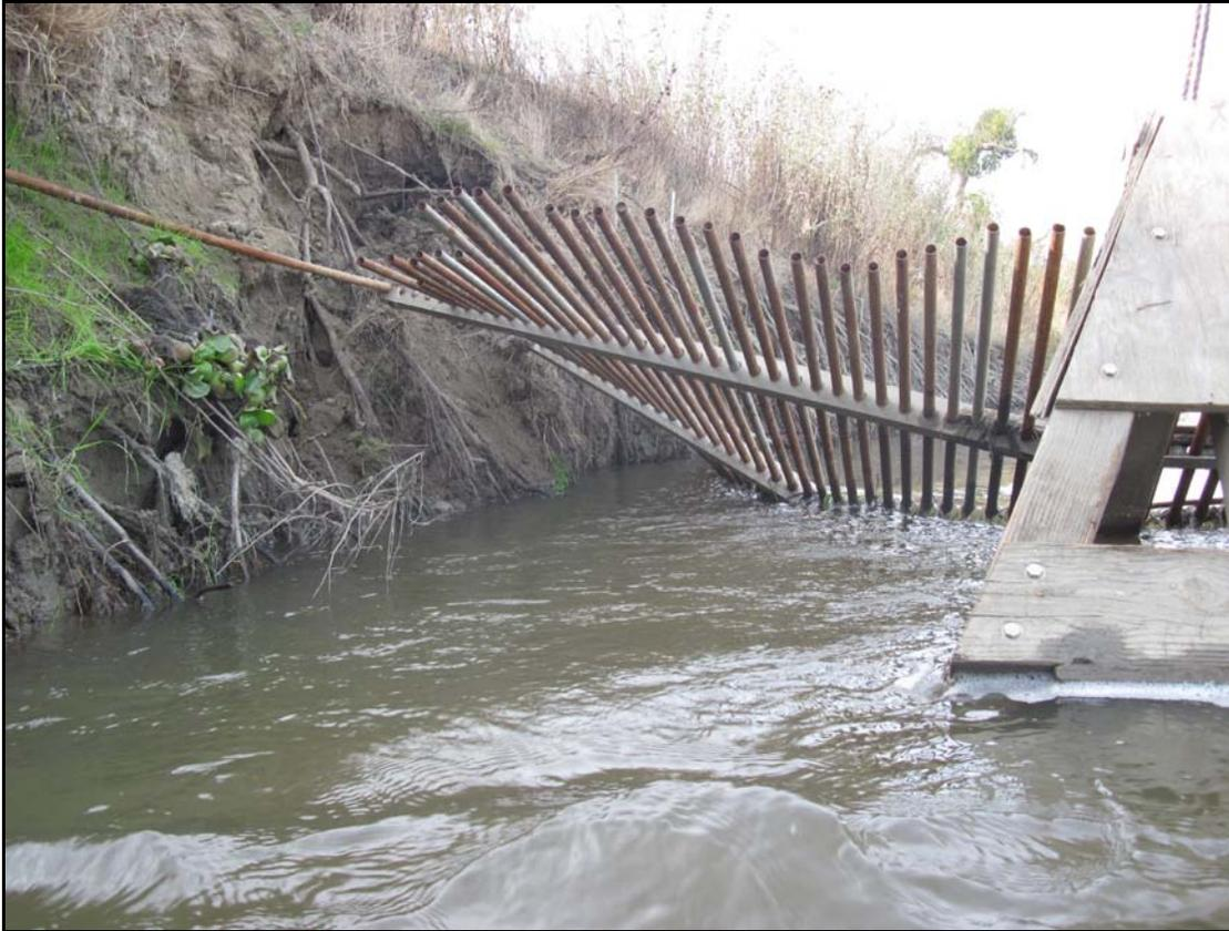
Figure 13.—Bank erosion and scoring causes holes in the barrier which may provide upstream passage at the Hills Ferry Barrier.
