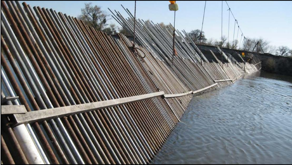
Figure 3.—Hills Ferry Barrier is a sliding pipe weir constructed of aluminum channel with 2.5-cm (1-in) holes that allow 1.9-cm (.75-in) electrical conduit to slide freely vertically in the corresponding holes and are pushed into the riverbed.
