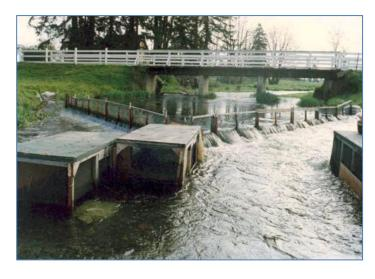
Temporary fish collection structures will include flashing lights and flagging to alert boaters. As appropriate, temporary fence weirs will include a removable panel marked with bright paint and signage to direct boaters for motorboat passage. Reclamation will place signage to alert boaters of the temporary fish collection structures.
